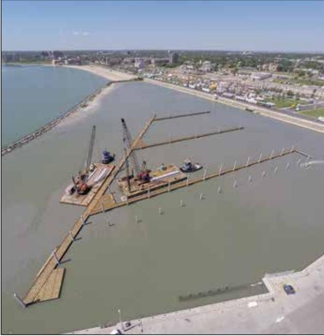
*The new docks, built by MEECO SULLIVAN, are floating wooden docks with 18-inch diameter concrete piling.*
