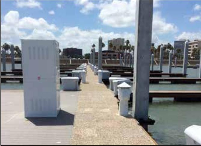
Instead of traditional wood decking, the marina installed three-foot concrete pavers that don't use galvanized screws, which corrode in the saltwater environment.
